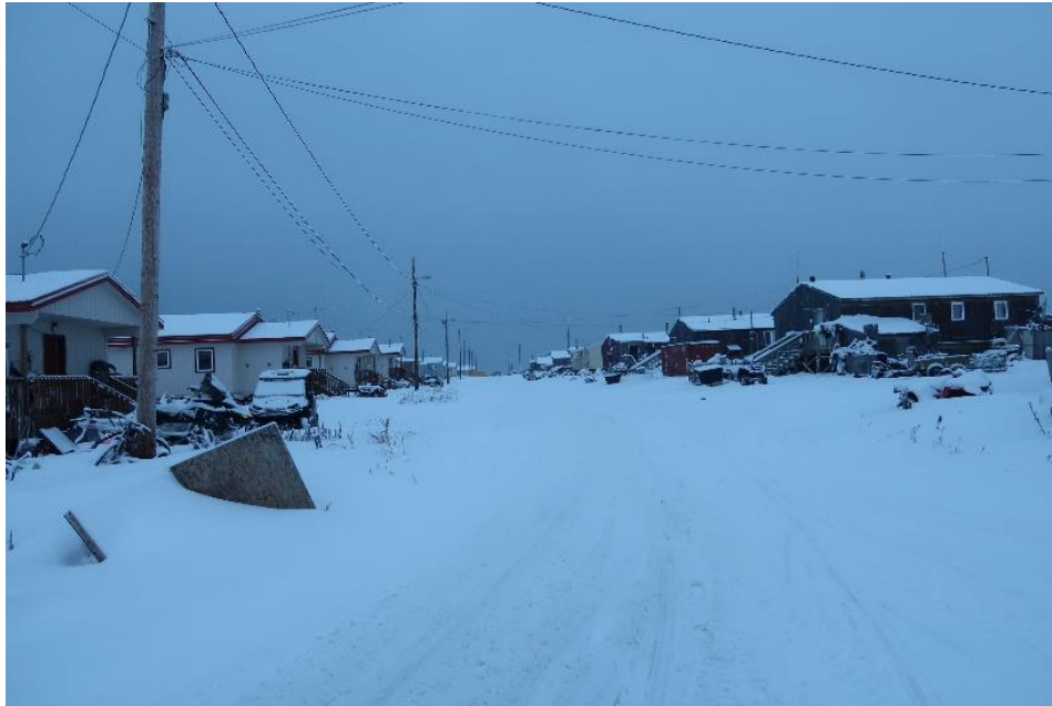
Figure 2. Shishmaref Main Street in November 2018.
