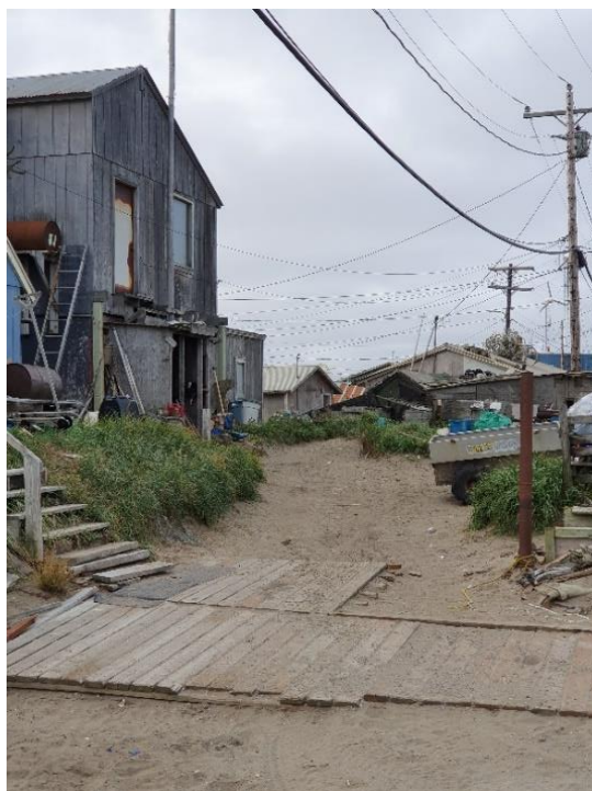
Figure 8. Shishmaref street view in August 2019.
