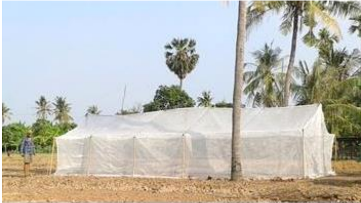
Figure 5: Participatory research led to the redesign of low net tunnels into a Nethouse structure farmers could enter and walk through.
